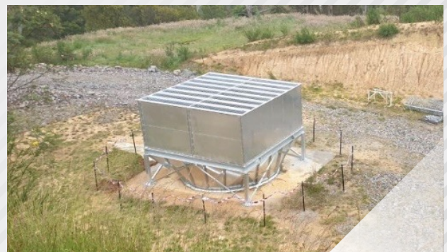
Final installation of the attenuator on the Dargues Mine ventilation fan
