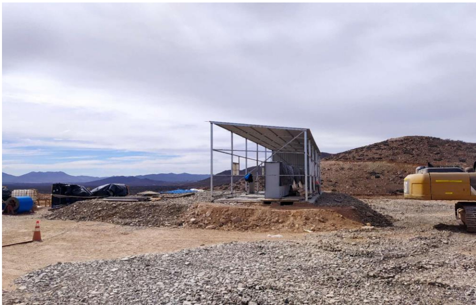
Figure 5: Power distribution room
