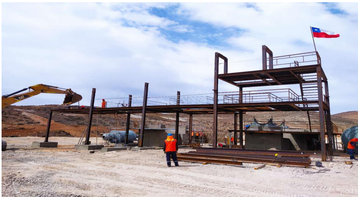
Figure 3: Installation of No. 1 and No. 2 ball mill operating platforms
