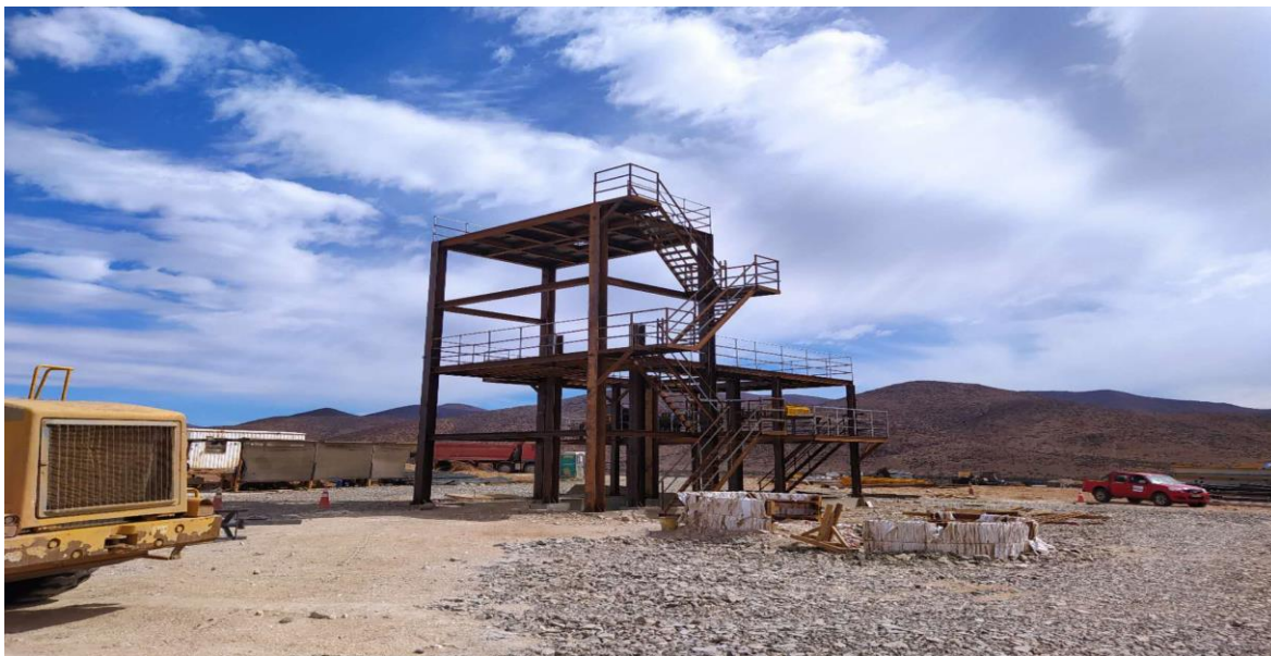
Figure 1: Screening platform and No. 3 belt conveyor
