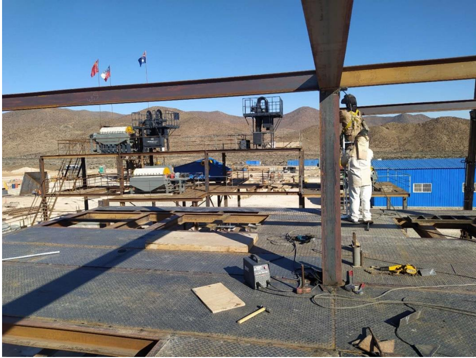
Figure 4: Construction work on new plant
