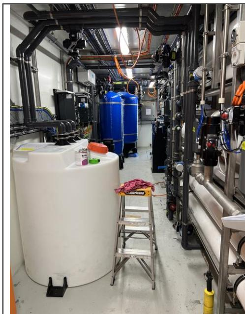
**Image 1) De.mem Containerized Membrane Based Water Treatment Plant**
