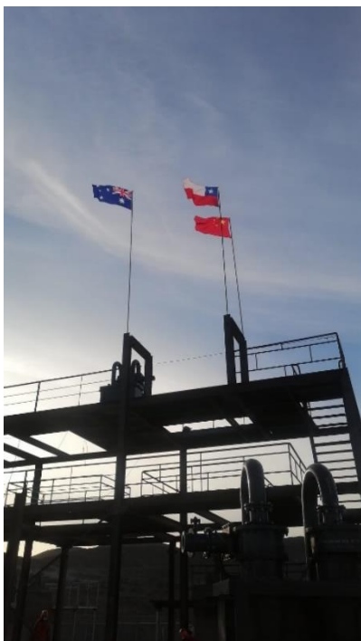
Figure 1: No. 1 and No. 2 ball mill operating platforms
