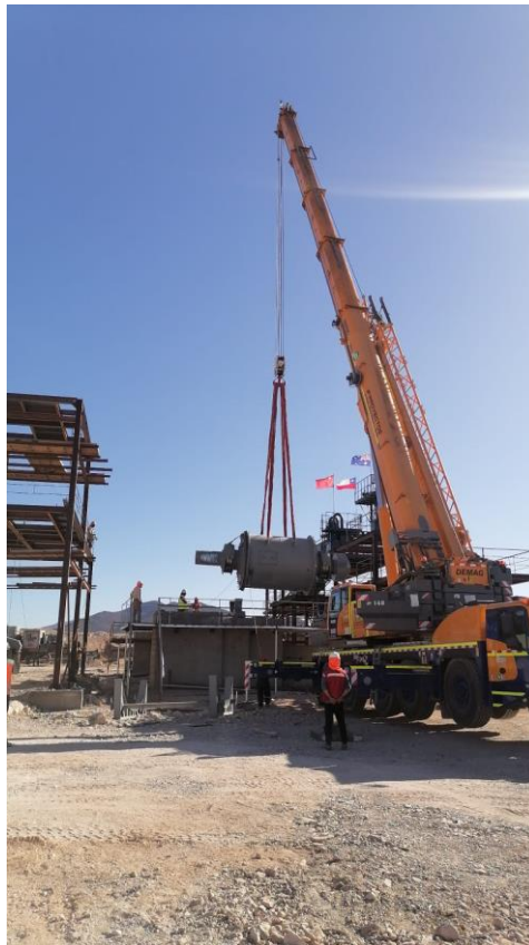
Figure 3: Installation of ball mill using high capacity crane
