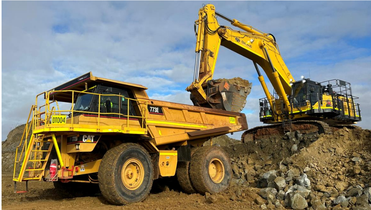
Figure 1: First load of waste from Greenfields loaded to complete TSF platform construction
