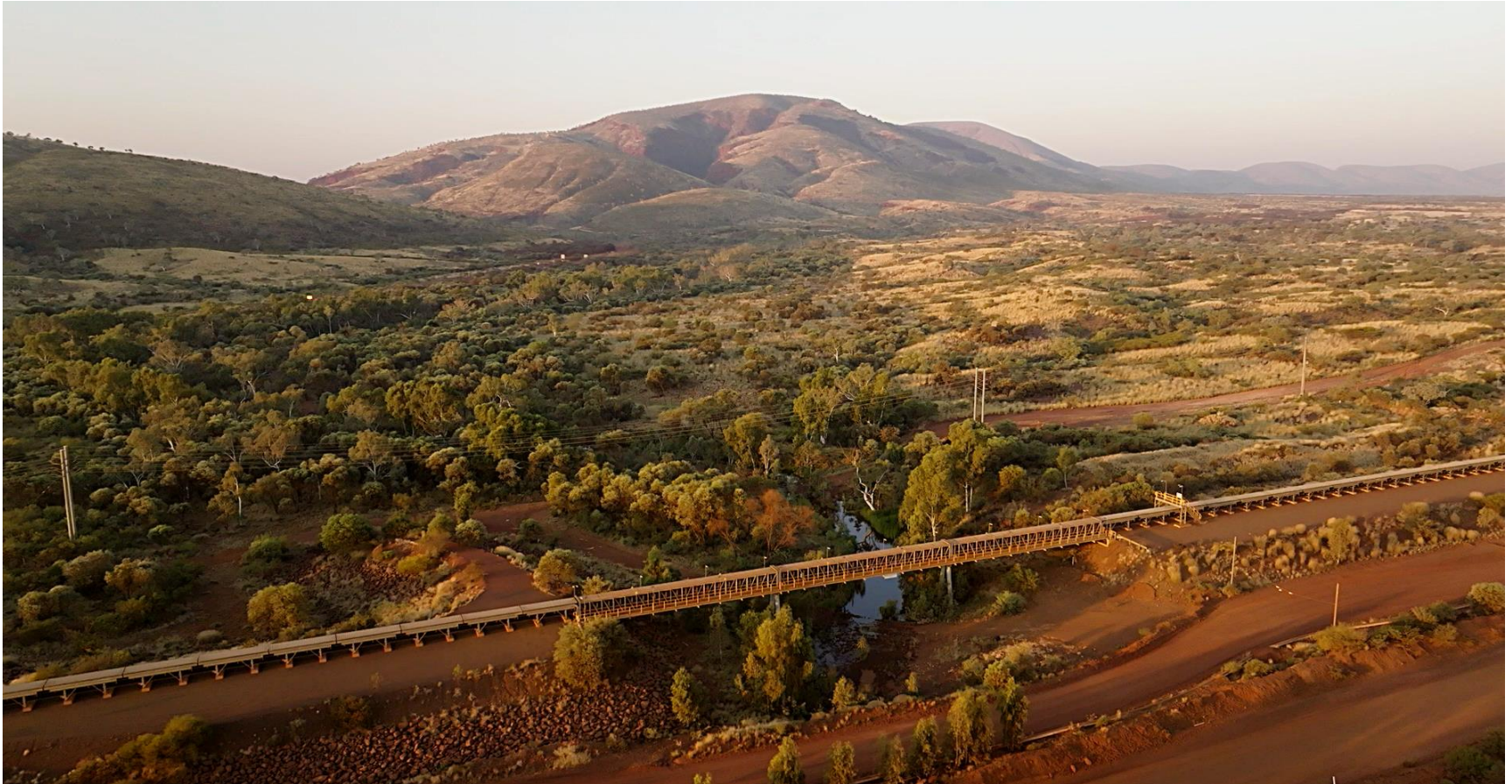
Rio Tinto's overland conveyor belt at the Western Turner Syncline mine, one of their longest conveyors in Western Australia's Pilbara region.
