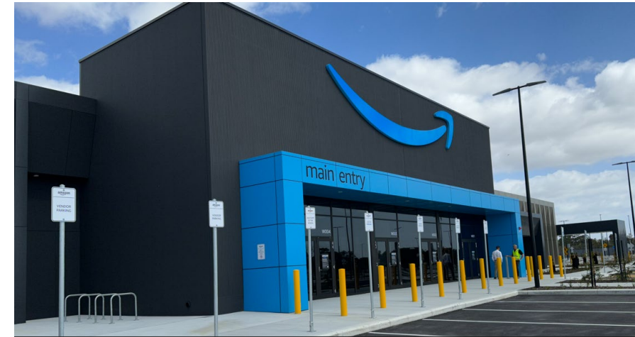
Amazon, Jandakot Airport industrial precinct, Perth WA
