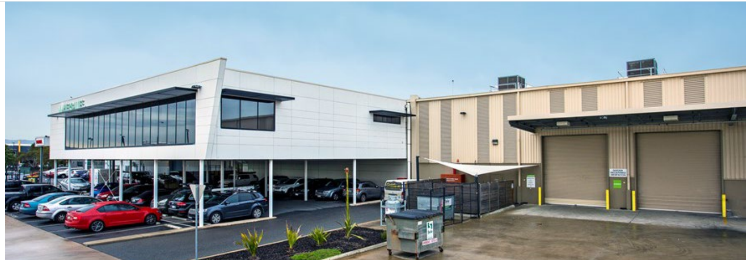
20 Butler Boulevard, Adelaide Airport SA
