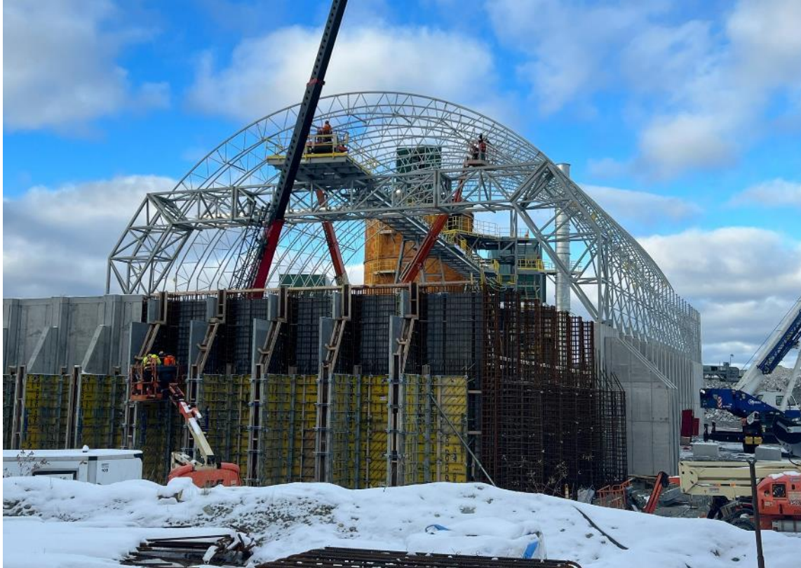
Crushed Ore Dome construction
