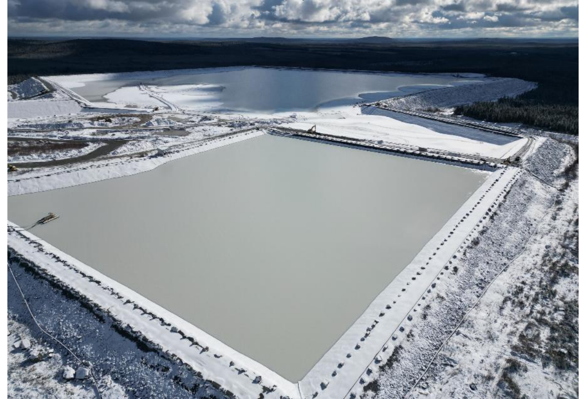
Tailings Storage Facility 1 project
