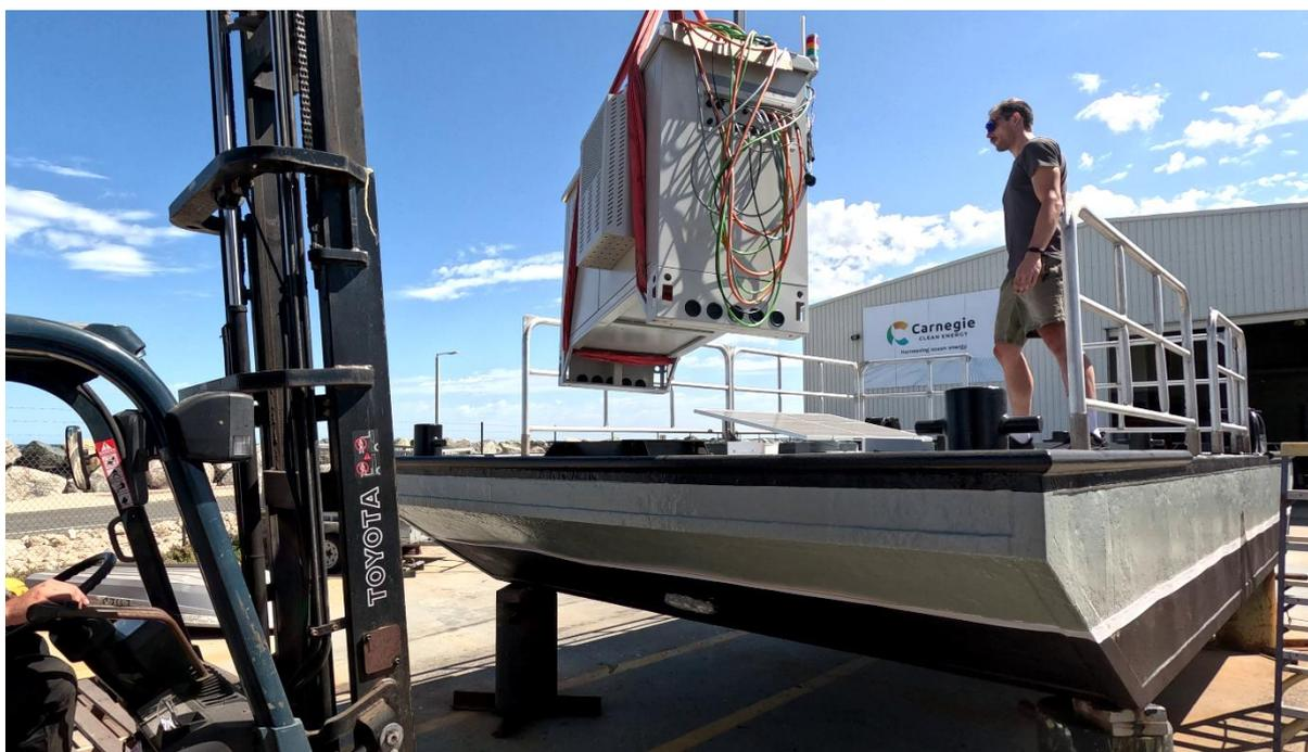
*Image: Placement of control system on MoorPower barge prior to PTO unit mounting.*
