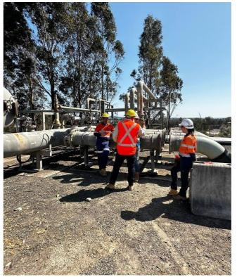
Gas is delivered to the CGP via the buried gas gathering system at low pressures to maximise well deliverability
