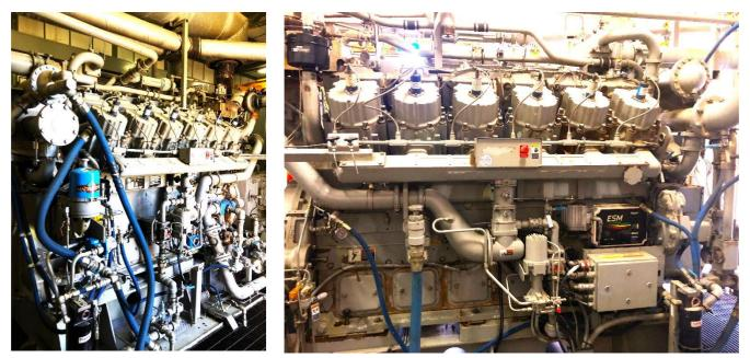
Part of the newly acquired RPGP - Low pressure gas is compressed to sales gas pressure using gas engine driven reciprocating compressors
