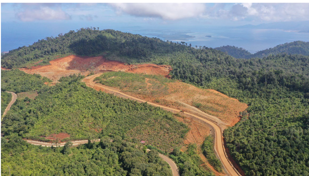
Aerial view of the rehabilitation of the Central Pit 1
