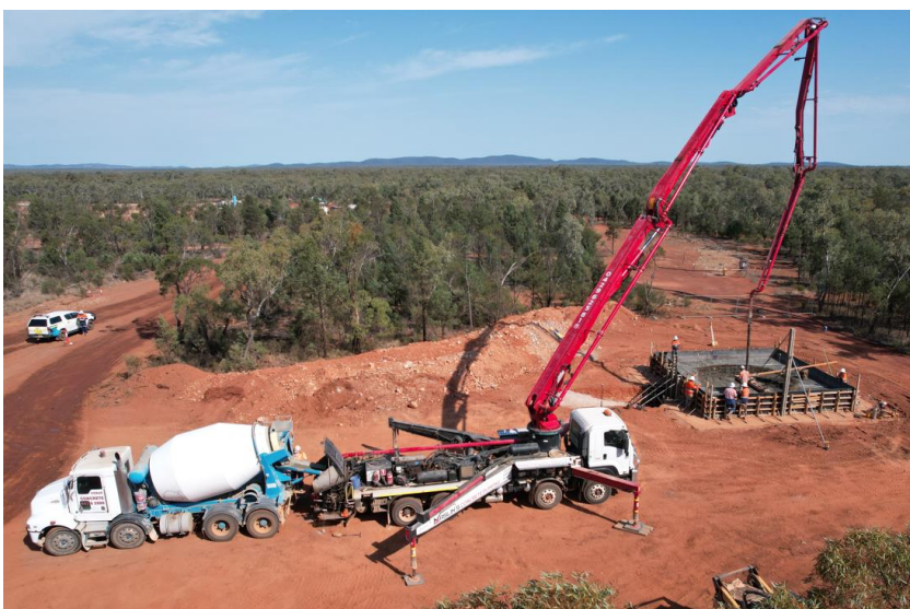
Image 2: Pouring of return air rise collar.
