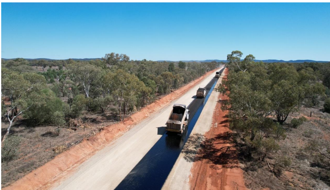
Image 1: Burthong Road sealing works in progress.
