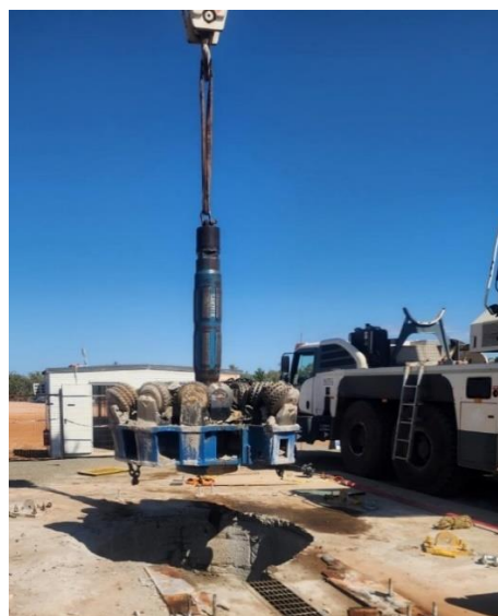
Image 3: Break through of egress rise shaft
