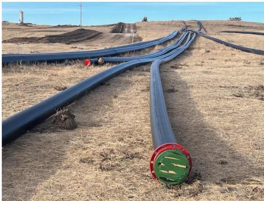
Figure 4 – Large diameter pipelines being prepared for MU-3
