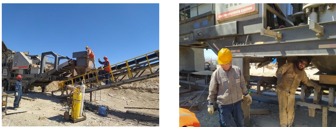
Figure 1: Installation of jaw crusher and coarse cone crusher
