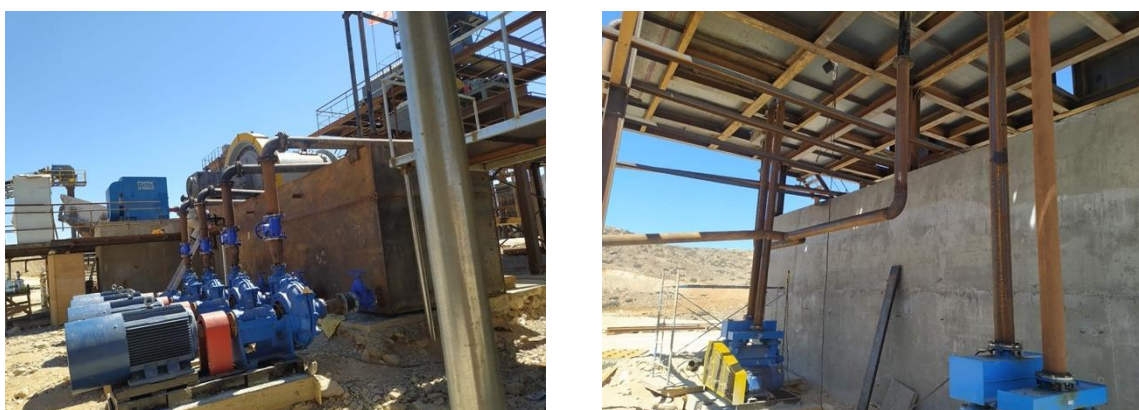
Figure 2: Other installation work included the filter and concentration magnetic separator
