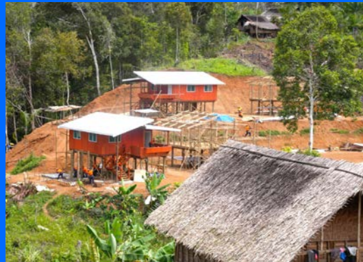
Pimaga teacher housing under construction
