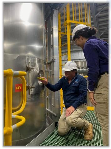
Stage 1 spray dryer under commissioning used for final processing of high purity alumina hydrate
