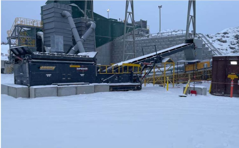
Figure 4 – Refeed System nearing completion
