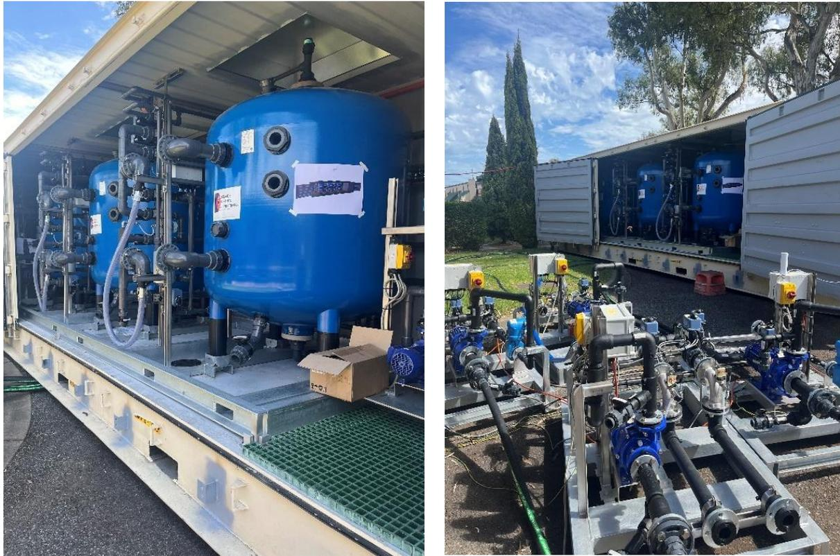
**Figure 3:** IX columns completed installation inside container. Pump skids in the foreground connected in readiness for Factory Acceptance Testing.
