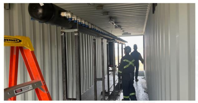
Figure 6: Installation of injection manifold at new Header House placed in MU-3
