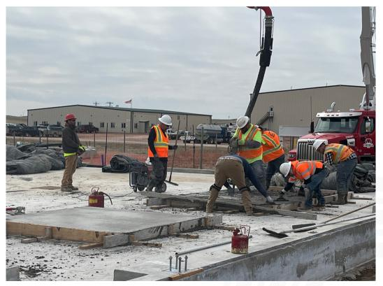
Figure 4: Foundation and tank pedestals poured for the Filtration Building (early April 2024)
