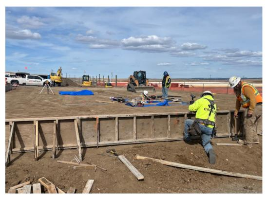
Figure 3: Preparing forms for a 250-cubic yard concrete pour (March 2024)
