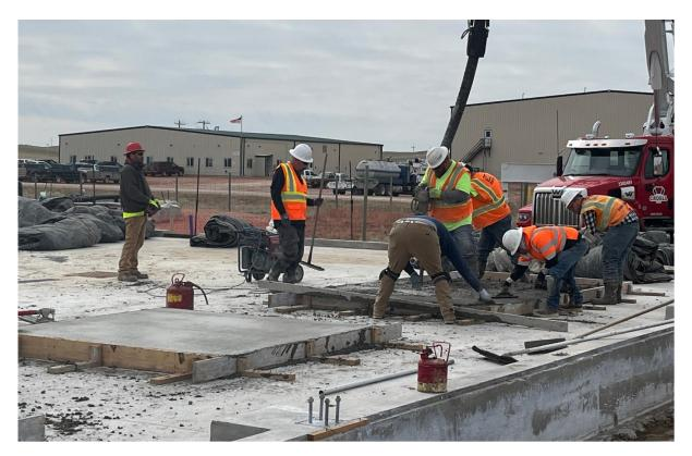
Figure 2: Foundation and tank pedestal concrete work for the filtration plant at Ross CPP
