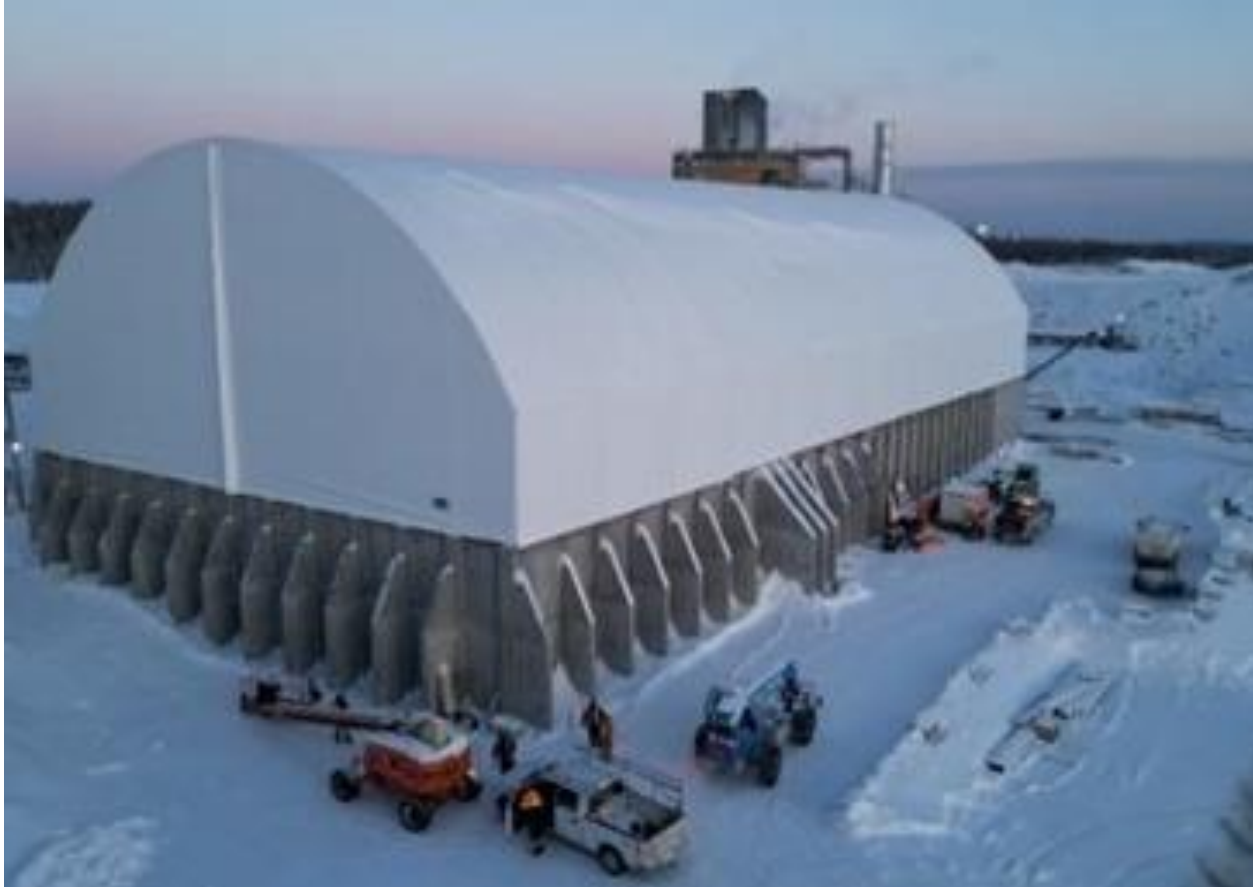
Crushed Ore Dome
