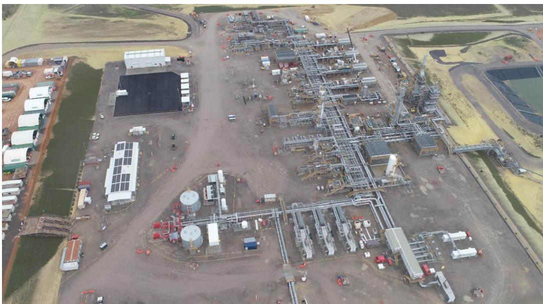
Waitsia Gas Plant during pre-commissioning
