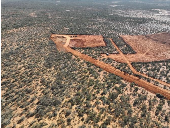
Figure 4: TSF4 thickener clearing works, now complete
