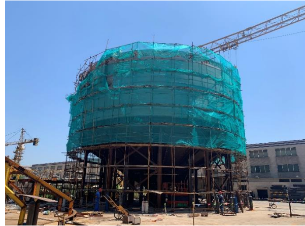
Figure 5: Off-site thickener fabrication
