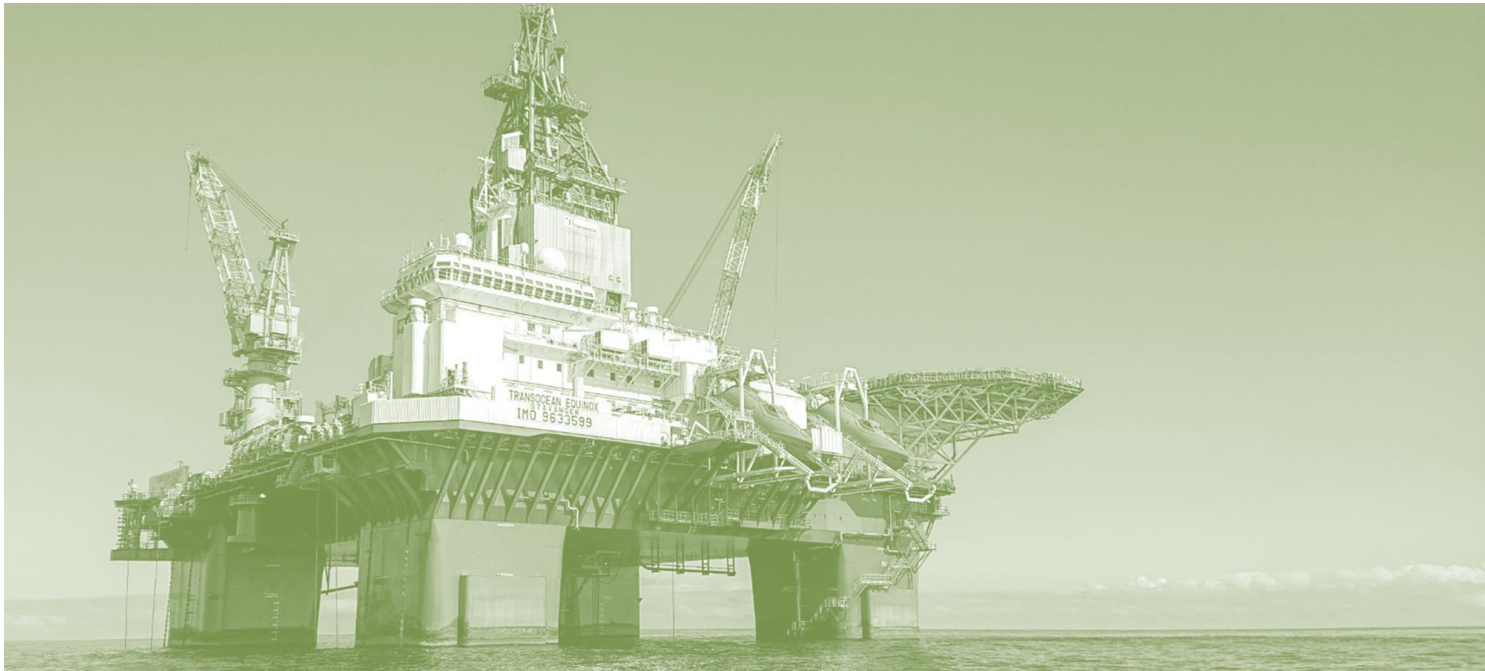
Figure 1: Transocean Equinox semi-submersible drilling rig
