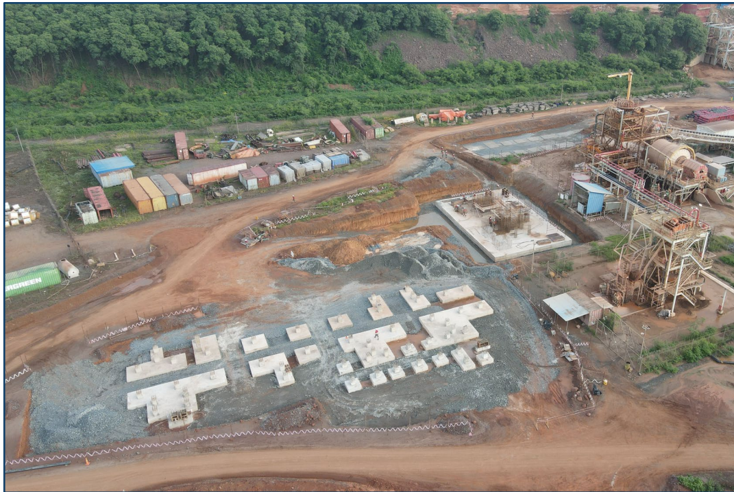
Ball mill and flotation area foundations
