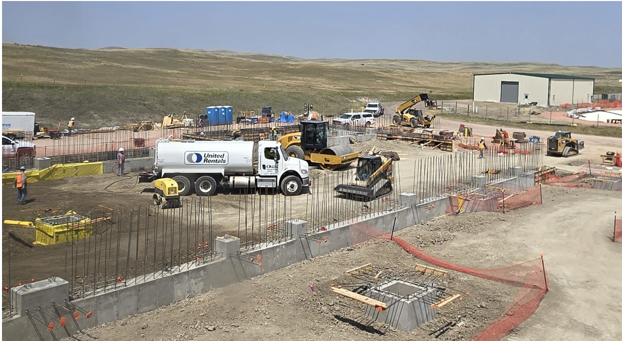
Figure 2: Concrete foundations at the Ross CPP expansion location
