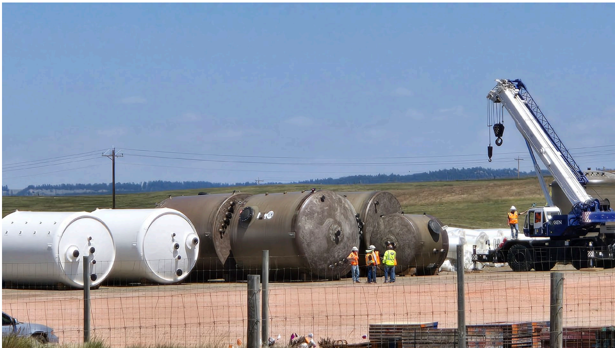
Figure 3: Process tanks for the plant expansion being received at Lance
