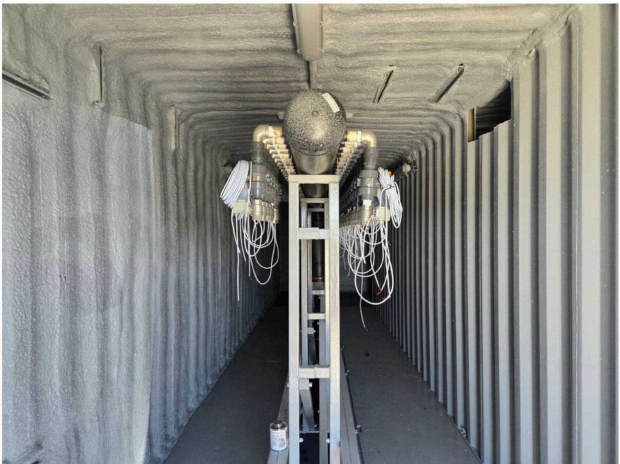
Figure 6: Preparation of MU-3, Header House 11 building interior
