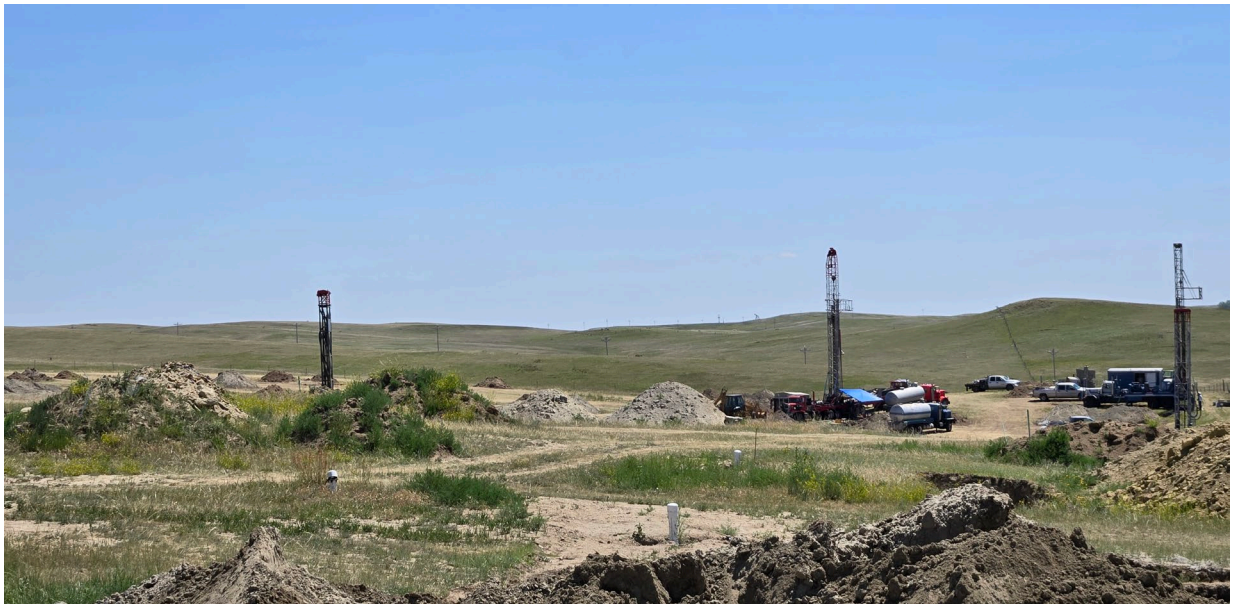
Figure 5: Active well installation at Mine Unit 3
