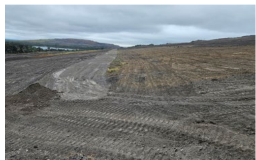
Early stages of the rehabilitation process at Peak Downs
