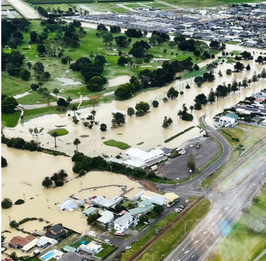
Flooding caused by Cyclone Gabrielle.
