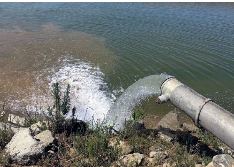
The new CBO-funded water pipeline for the Hungry Hollow District, California
