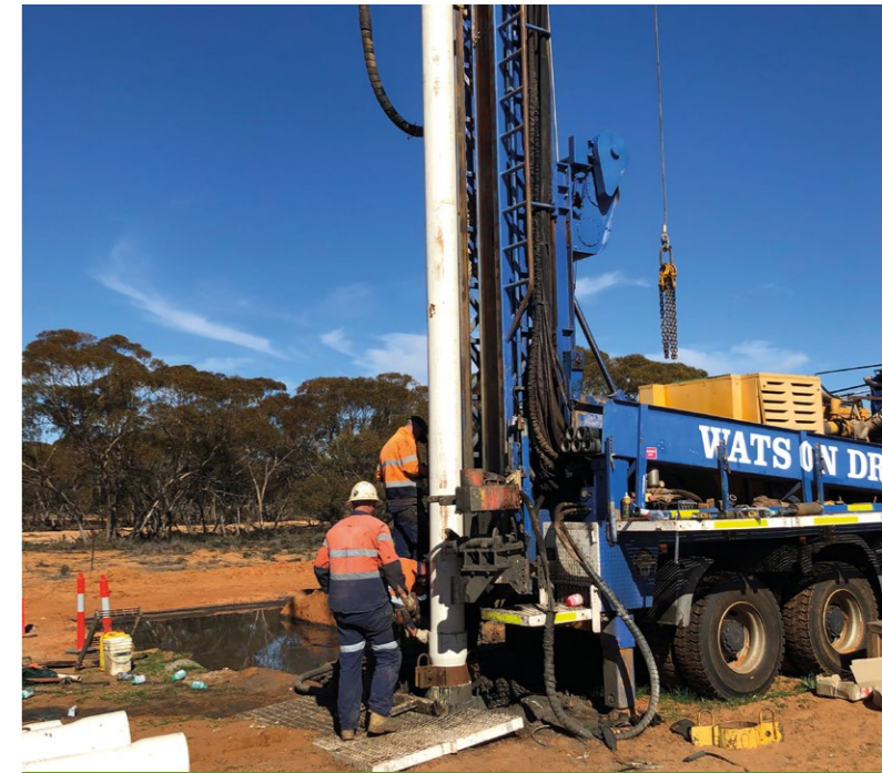
Drilling for groundwater at Boundary Bend
