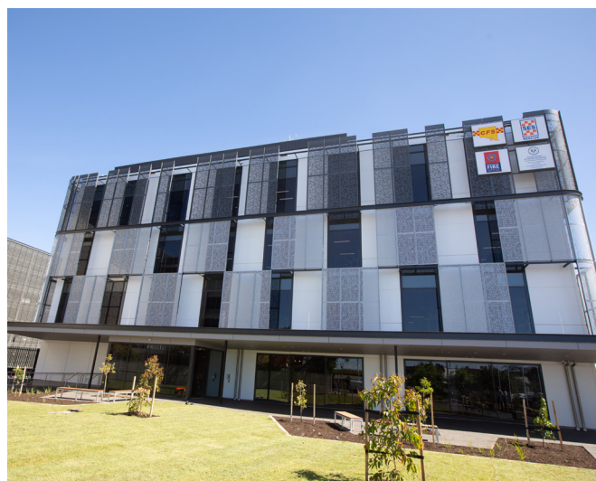
South Australian Emergency Services State Control Centre, SA
