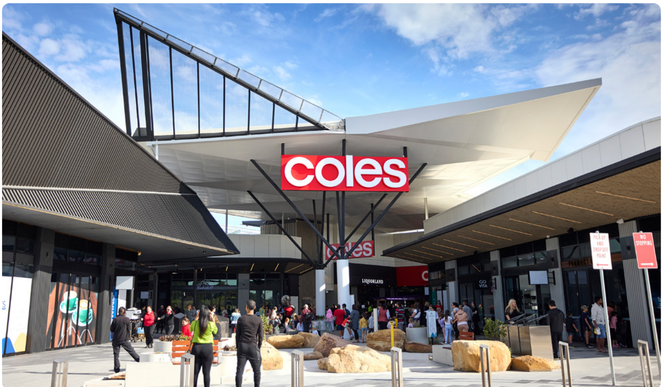
Pictured: Newly opened Coles Box Hill, NSW.
