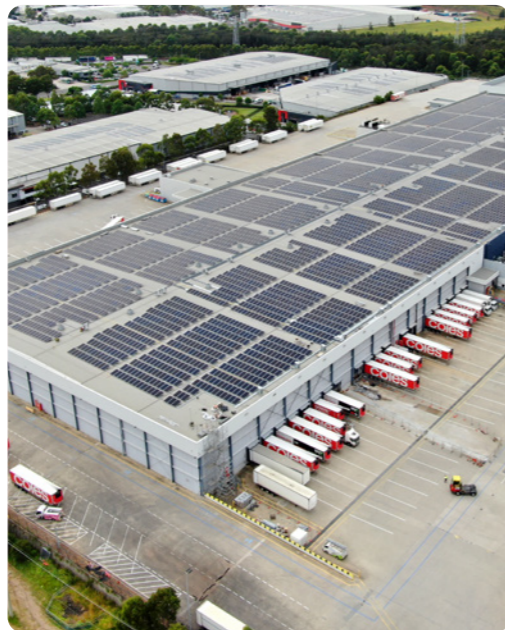
Pictured: Coles’ distribution centre in Eastern Creek, NSW, which is included in the 3-star Green Star Performance certification.
