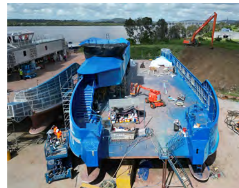
Southern Moreton Bay Island vessels under construction
