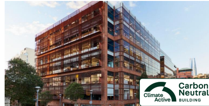
19 Harris Street, Pyrmont, NSW
