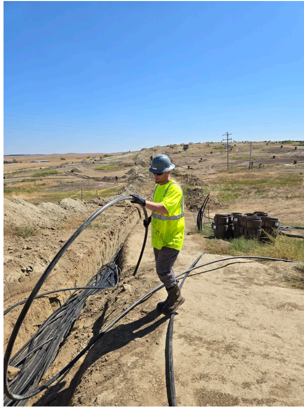
Figure 4: Connecting HH-11 wells to the header house building
