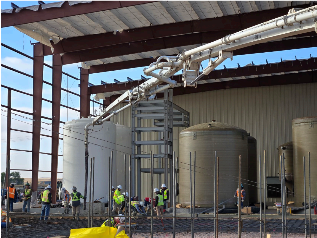
Figure 2: Concrete slabs being poured at the Lance process plant
