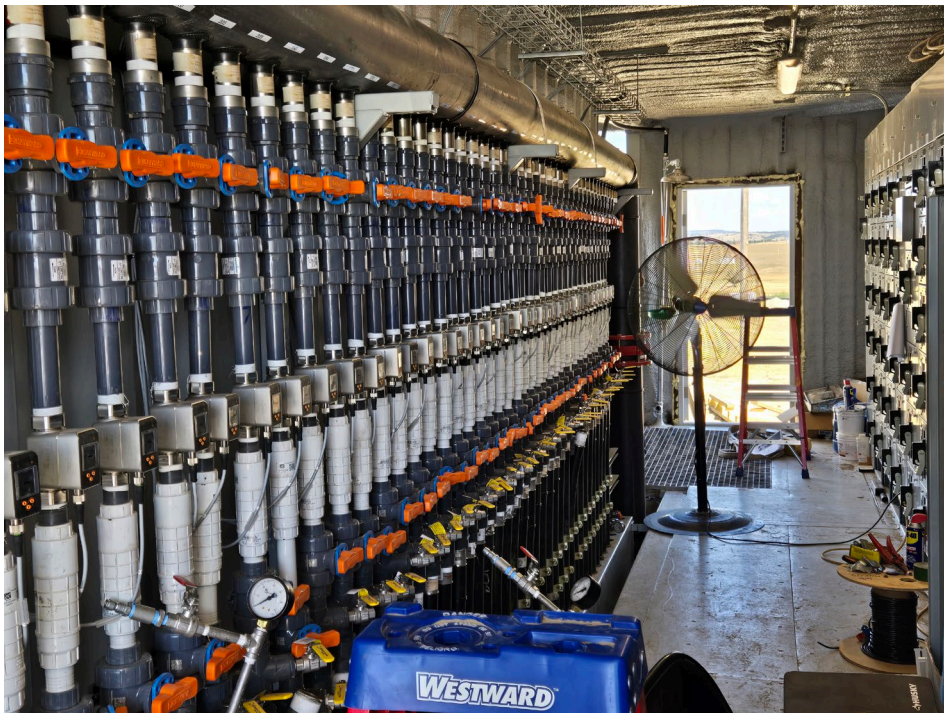
Figure 5: HH-11 interior under construction in August 2024
