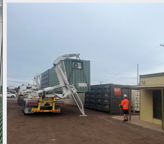
Delivered to site
