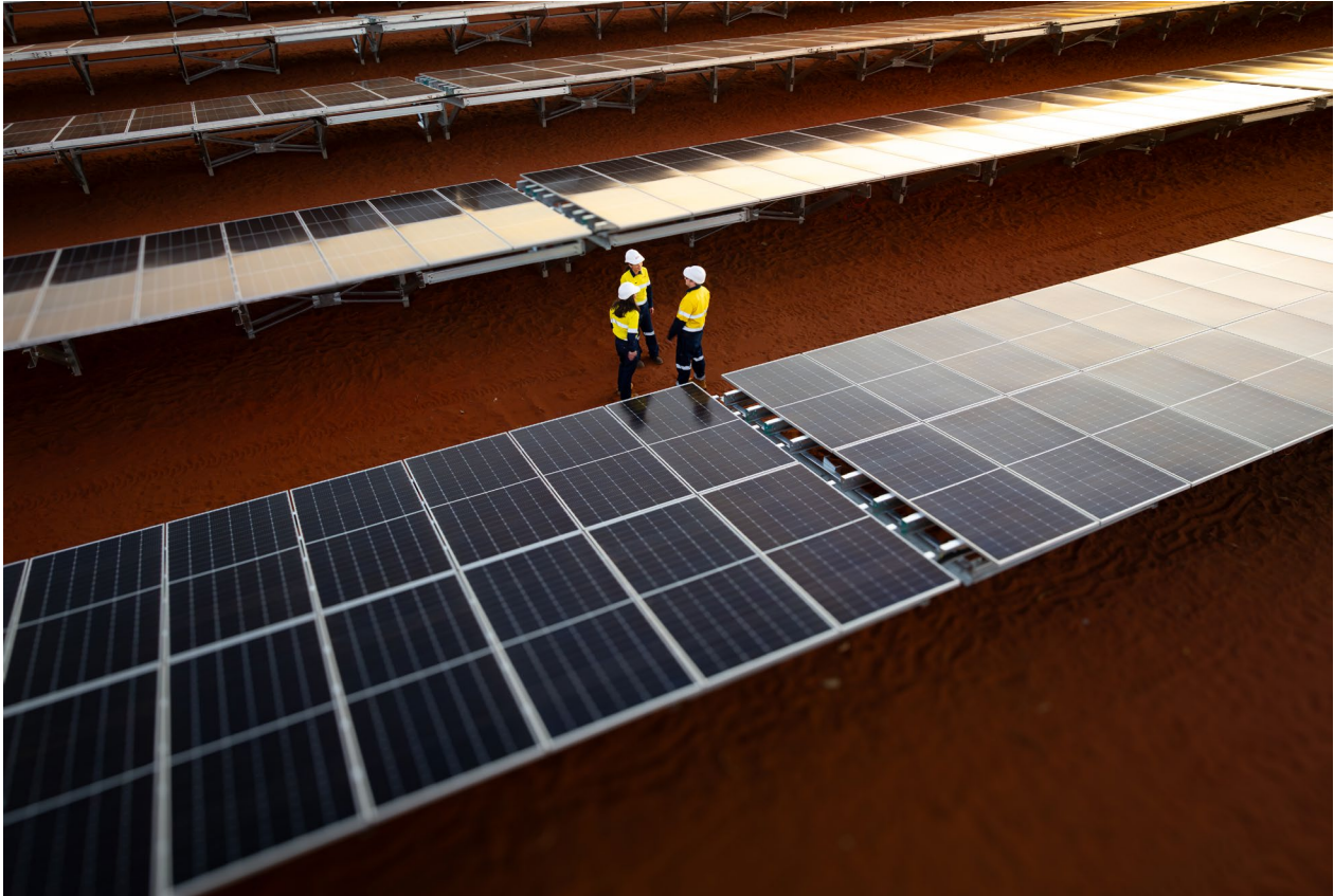
Port Hedland Solar Farm (under construction), WA ▲
