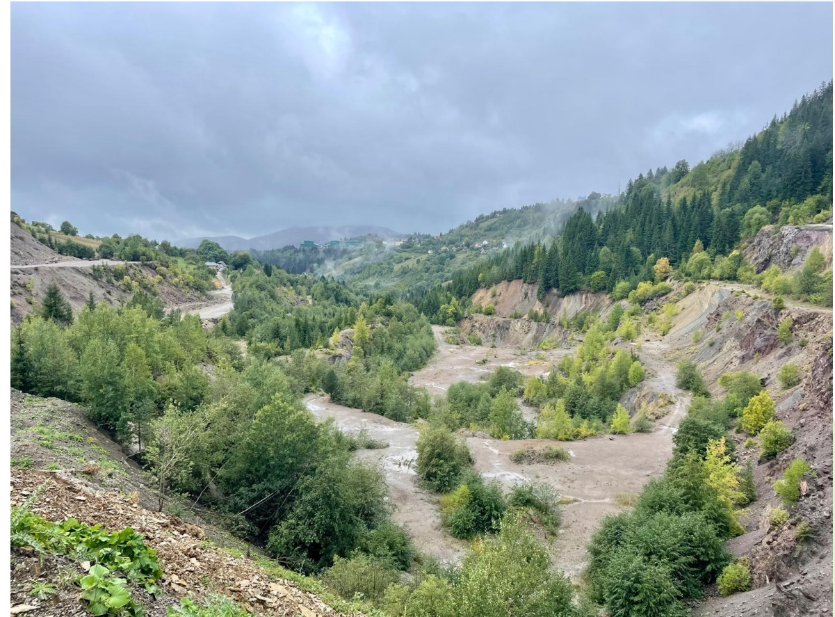
Veovaca Tailings Storage Facility
