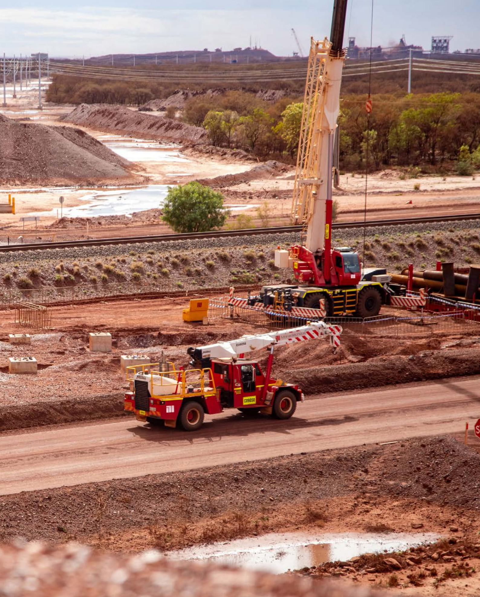
Construction of Fortescue's Christmas Creek overland conveyor, Pilbara region, Western Australia.
