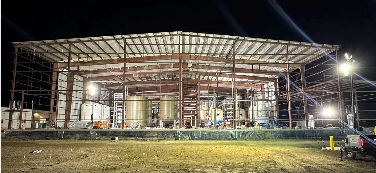
Figure 2: Lance Process Plant expansion showing interior equipment installation
