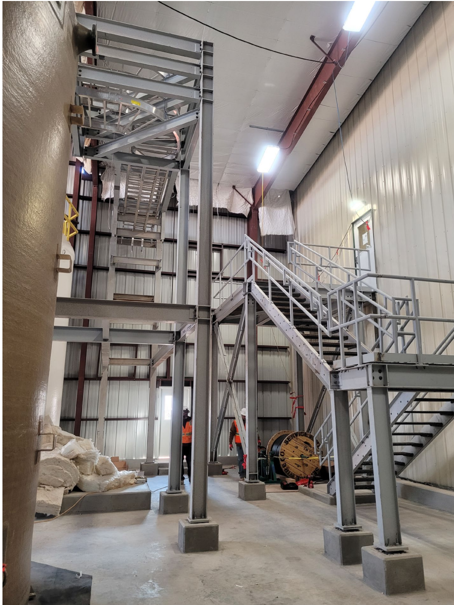
Figure 4: Interior photo of new CPP building construction progress
