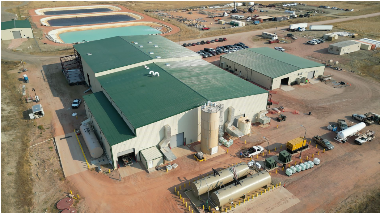
Figure 1: Drone image of Lance Project Facilities on 09-October 2024
