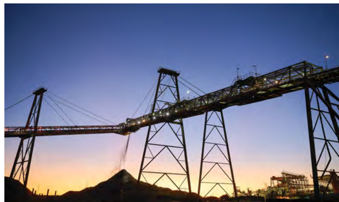
Ernest Henry processing plant and stockpile
