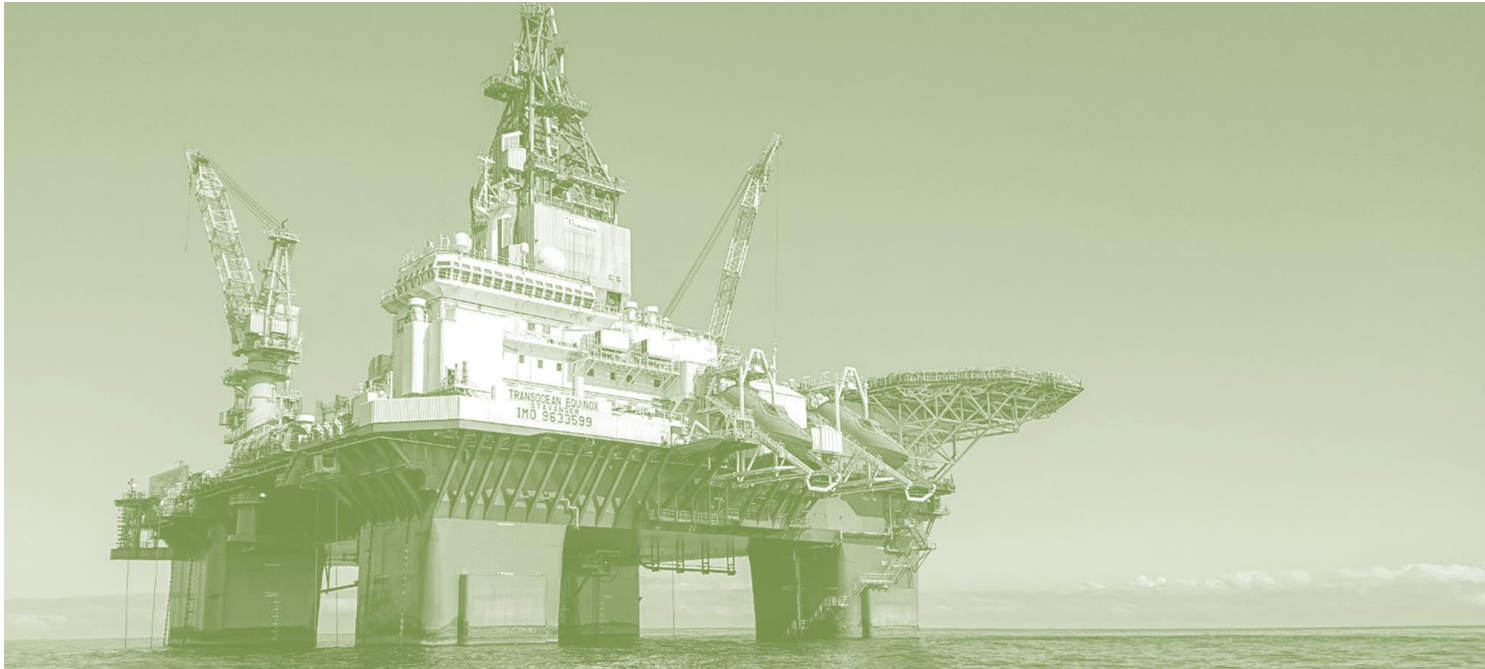
Figure 1: Transocean Equinox semi-submersible drilling rig
