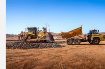
Perdaman Project Bulk Earthworks
