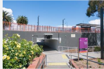
Gippsland Line Upgrade
