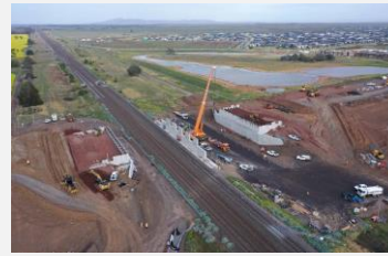
Ison Road Overpass
