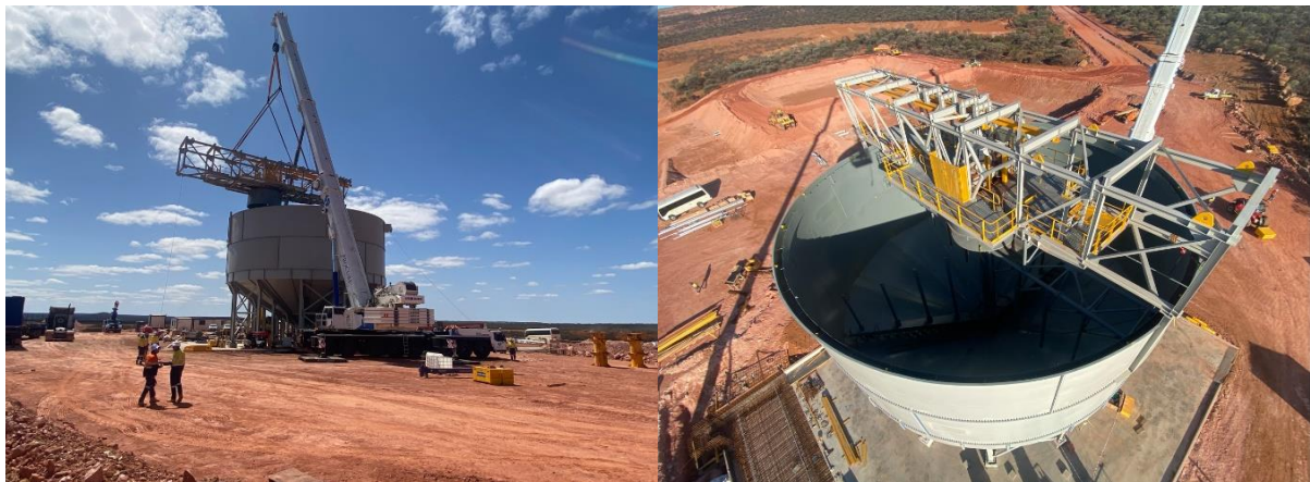
Figure 7: TSF 4 thickener assembly
