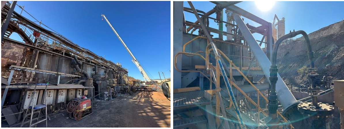
Figure 9: Repurposing of the processing plant as an interim water treatment plant
