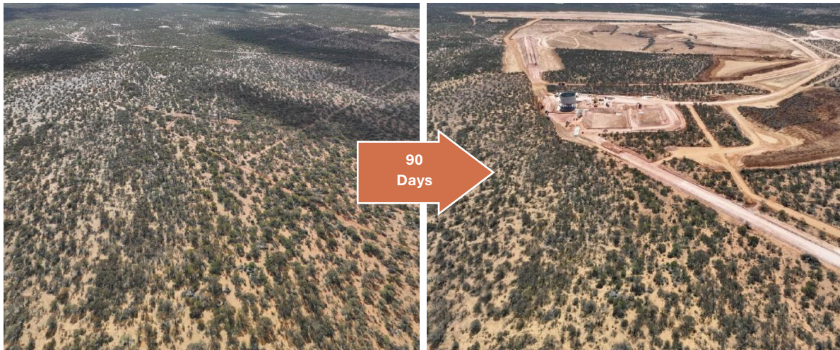
Figure 6: TSF 4 project, 90 days of progress
