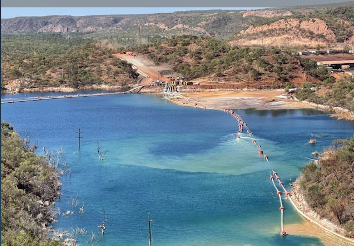
MCD water treatment, using recently commissioned MCD water treatment infrastructure
