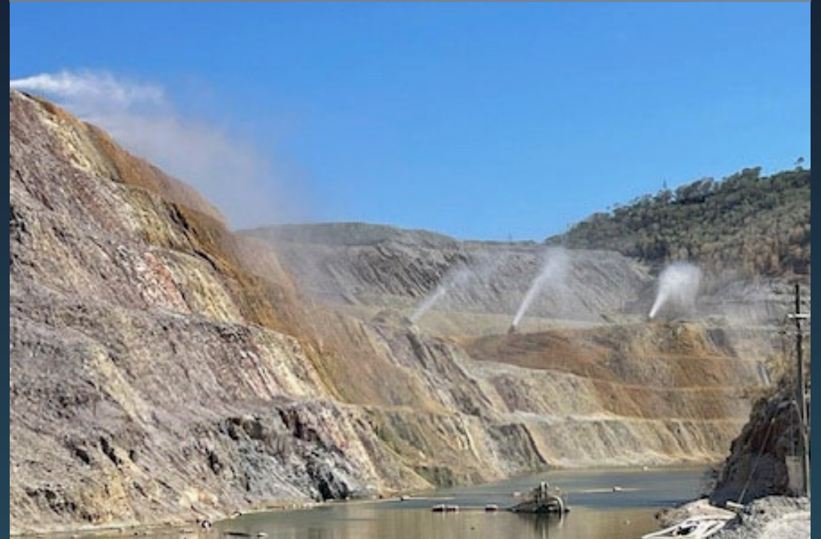
Mechanical evaporators at Esperanza Pit ('EPit')
