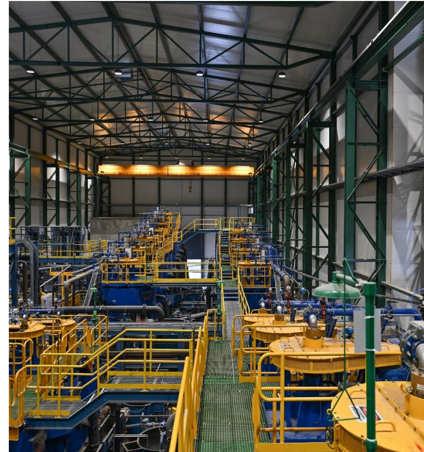
Vares Processing Plant, Aug 2024
