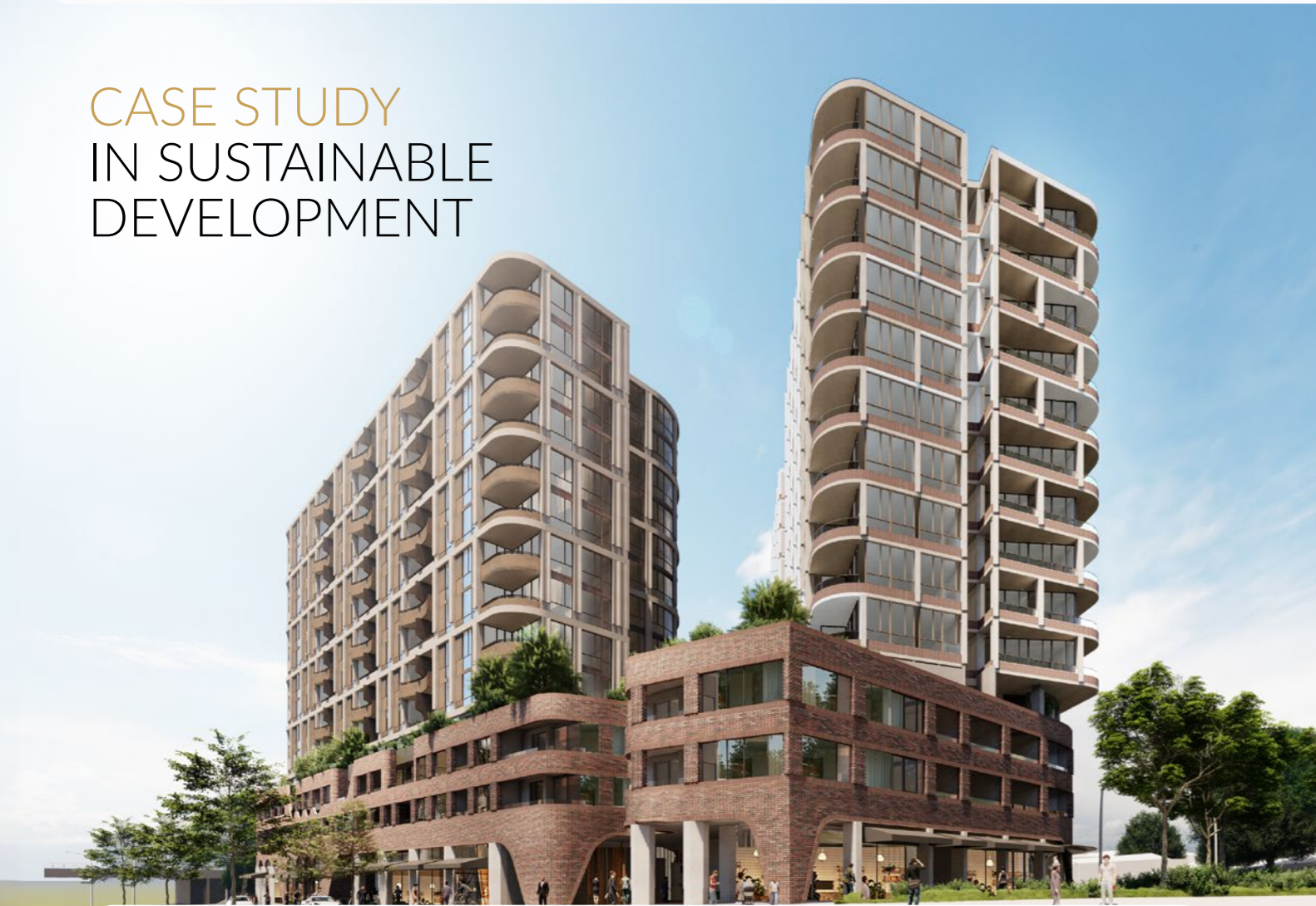
Caulfield Place Precinct 3 West
