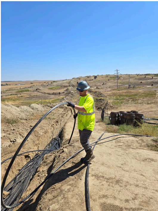
Figure 5: Connecting HH-11 wells to the header house building
