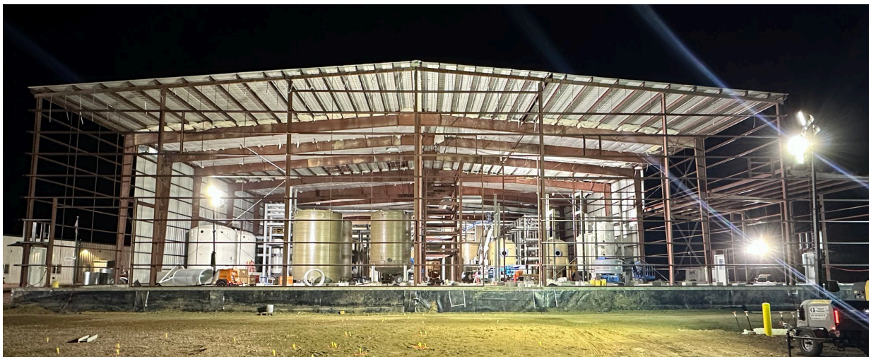
Figure 2: Expansion construction at the Lance Central Processing Plant
