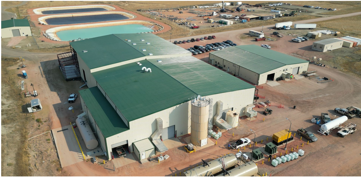
Figure 1: Peninsula's Lance Uranium ISR Process Facilities in Wyoming, USA
