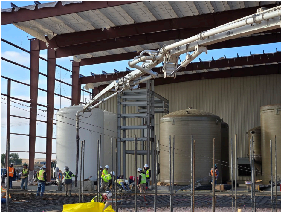
Figure 3: Concrete slabs being poured at the Lance process plant expansion
