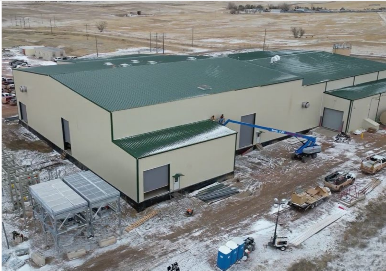
Figure 1: The Ross Central Processing Plant under construction, early November 2024
