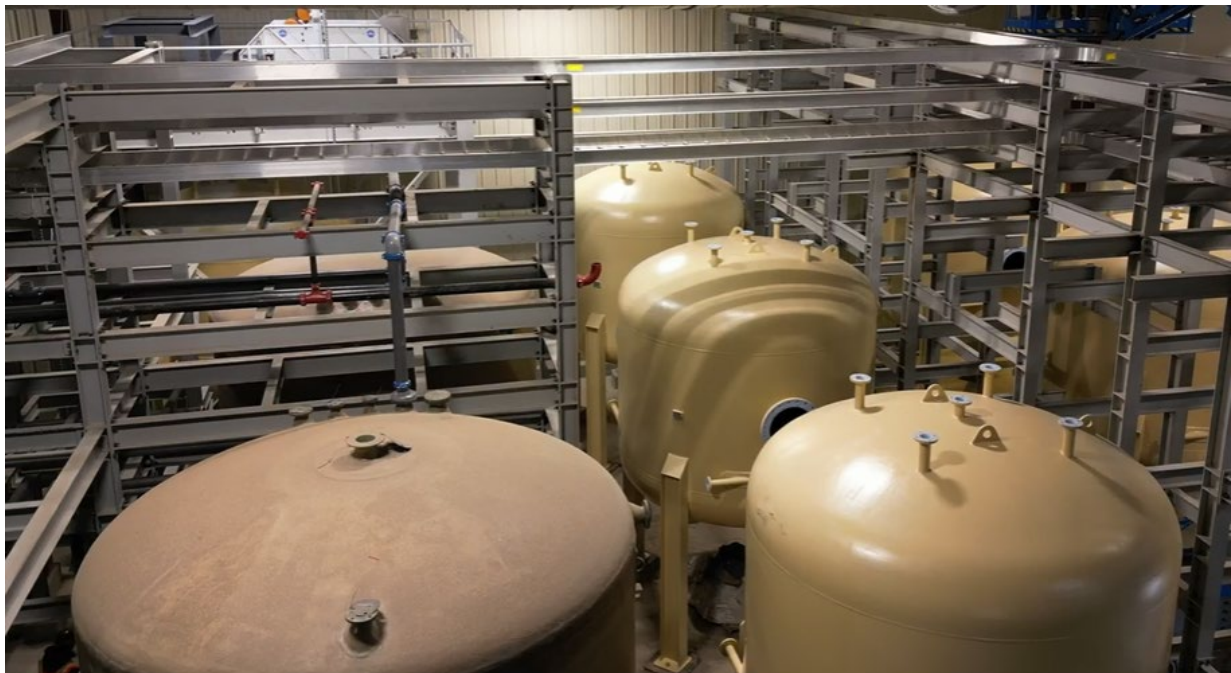
Figure 2: Structural steel and Ion Exchange systems under construction inside the CPP
