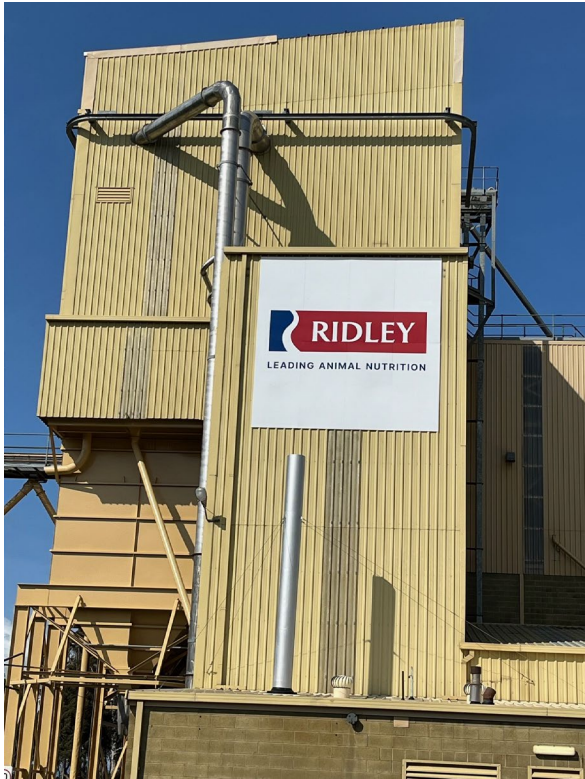
Carrick feed mill, TAS
